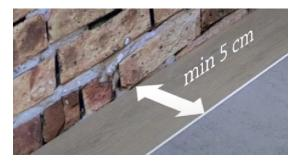
Normally the minimum panel width must not be less than 5 cm, and plank end joints must be staggered by at least  $\frac{1}{4}$  of the plank length.
